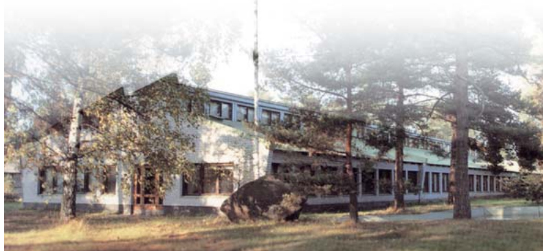
Helkama cable factory in Hanko, Finland.
