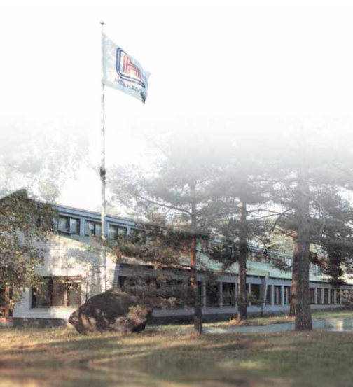
Helkama Factory in Hanko, Finland Marine cables and industrial cables
